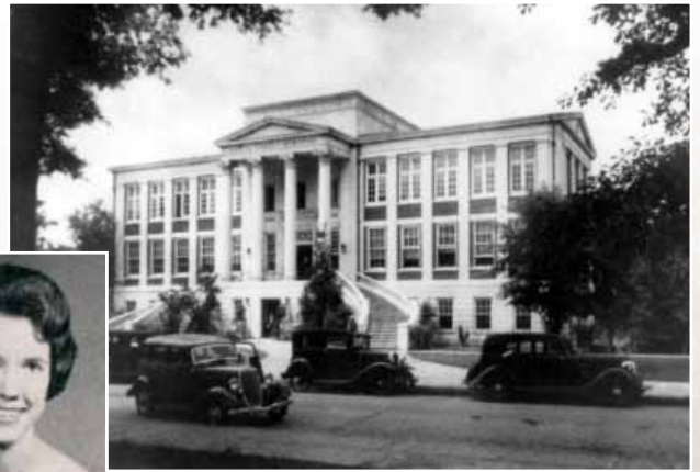
Jeanice Kirkland (inset in 1962 and below) and Carmichael Hall in the 1930s
