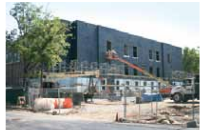
Renovating Foster Auditorium
