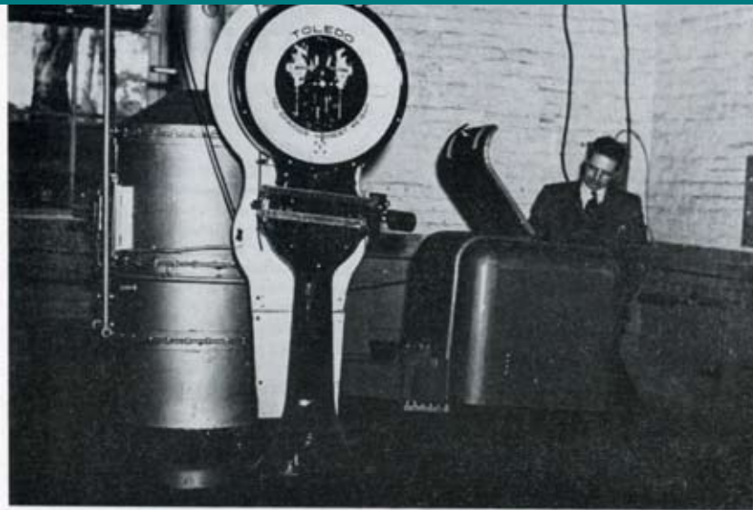
Mr. James R. Cudworth, director of the Mine Experiment Station and Chairman of the Research Committee, examines a stoker furnace unit used in a performance study for domestic stoker fuels of coals from certain Alabama fields.
